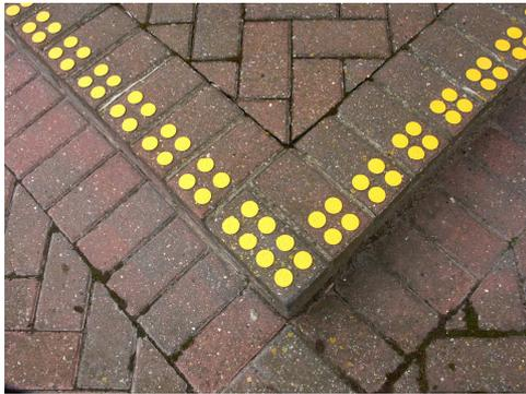
TreadSafe® abrasive coated stainless steel discs are specifically designed to provide a robust anti-slip solution for prestigious public access areas where an aesthetically pleasing appearance is a priority.
